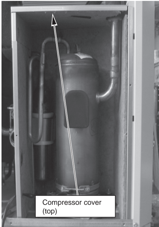
4. Remove the compressor cover (top).
